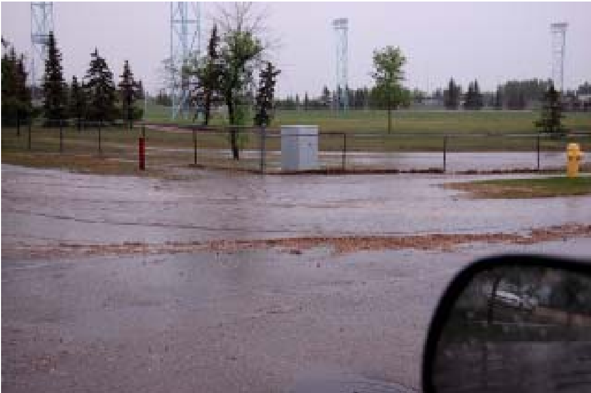
Photo 3.2: Major drainage system overflow from Mount Pleasant Drive to Kinsmen Park dry pond in June 5, 2007 storm.
