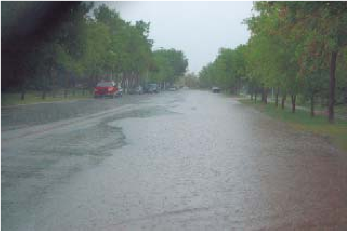
Photo 3.1: Major drainage system flowing to top of curb on Marler Drive in the June 5, 2007 storm.
