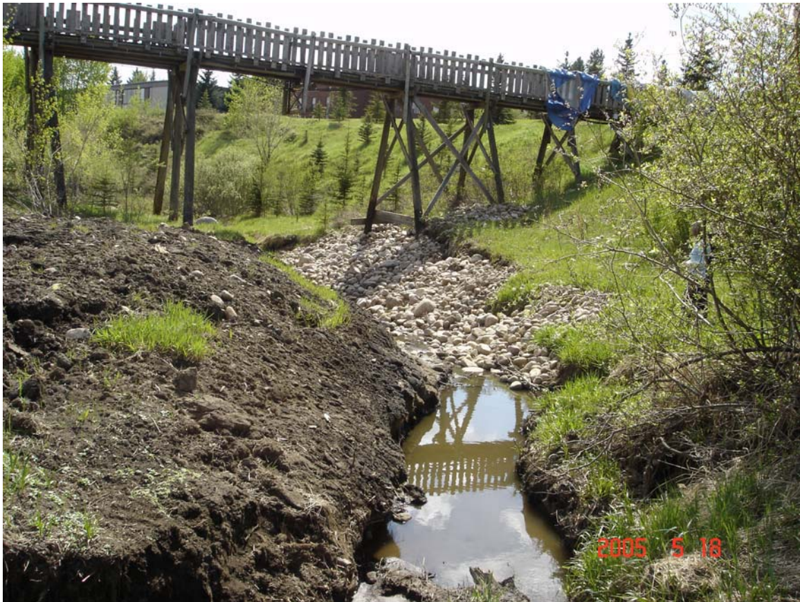
Photo 3.4: Bank riprap placed near the footbridge in Augustana College.
