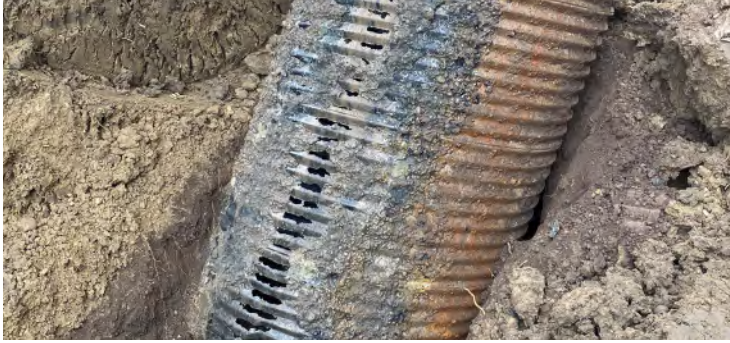
Storm main pipe beginning to fail (notice all of the holes)
