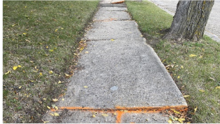
Faulting Hazard due to roots
