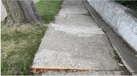
Faulting Hazard due to roots
