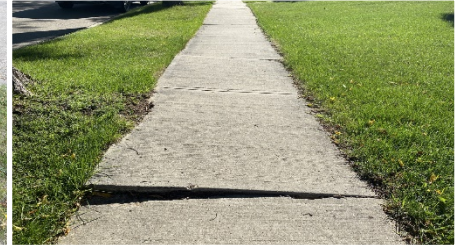
Faulting Hazard due to roots
