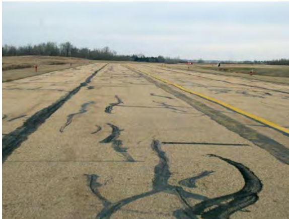
The airside pavement surfaces are approaching 20 years of service, exceeding the typical service life.
